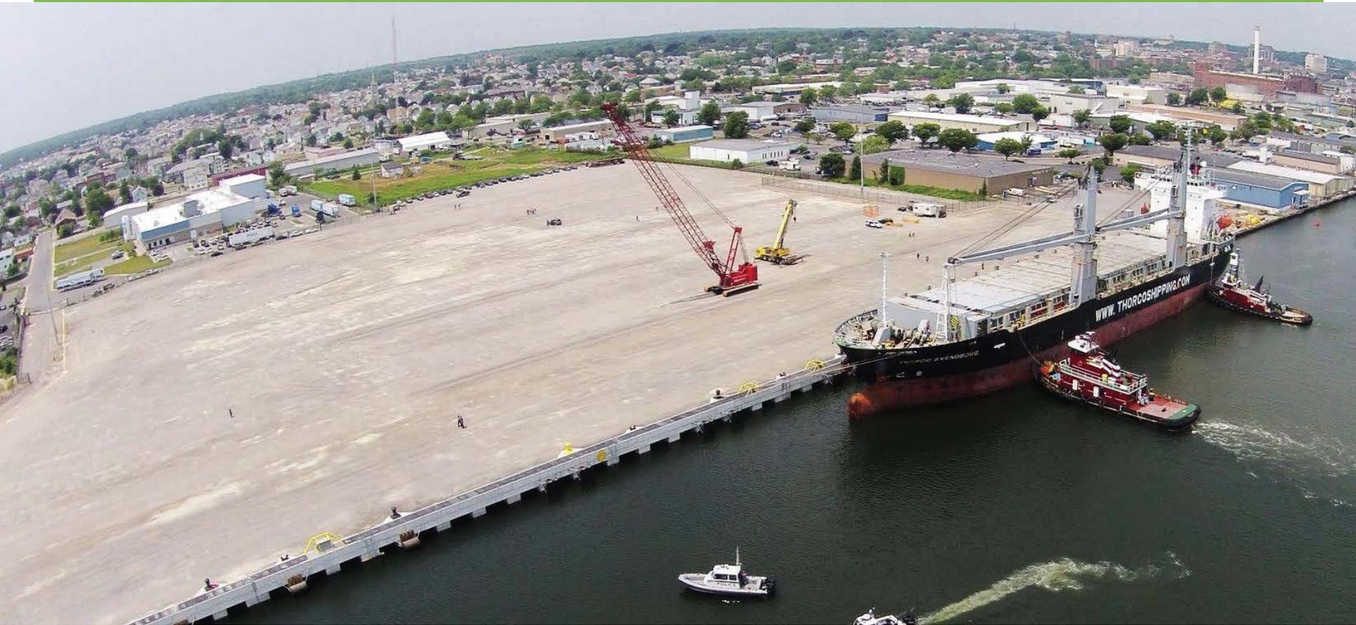
The state of the art 26-acre facility has a 1,200 foot quayside and a 300-foot wide navigational channel dredged to -30 feet. The site has the ability to sustain uniform loads of 4,100 pounds per square foot and concentrated loads of 20,485 per square foot.
