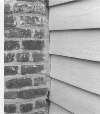
Figure 8. Appropriate mortar mixes should be used when masonry repairs are undertaken. In this case, a soft lime based mortar is used as an infill between the brick and wooden elements. When full repairs are made during the restoration phase, this soft mortar can easily be removed and missing bricks replaced.
