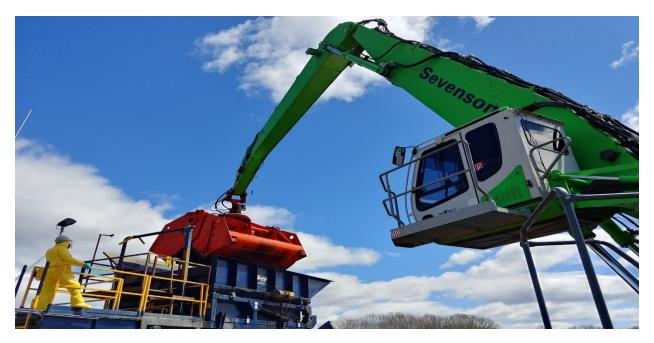
(Loading contaminated sediment for processing from precision dredging of Cable Crossing segment of the Acushnet River performed Fall 2017 to Spring 2018)
