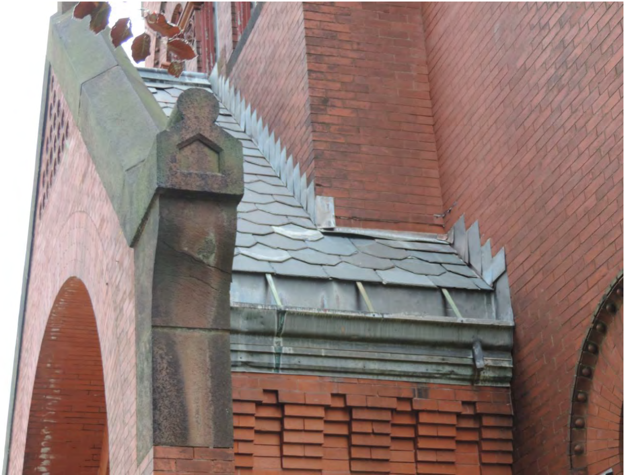
Rogers missing slates lifting flashing
