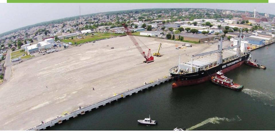
The state of the art 26-acre facility has a 1,200 foot quayside and a 300-foot wide navigational channel dredged to -30 feet. The site has the ability to sustain uniform loads of 4,100 pounds per square foot and concentrated loads of 20,485 per square foot.
