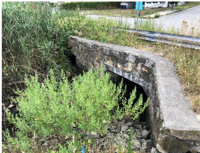
Image 2- Existing Headwall at Sycamore Street
