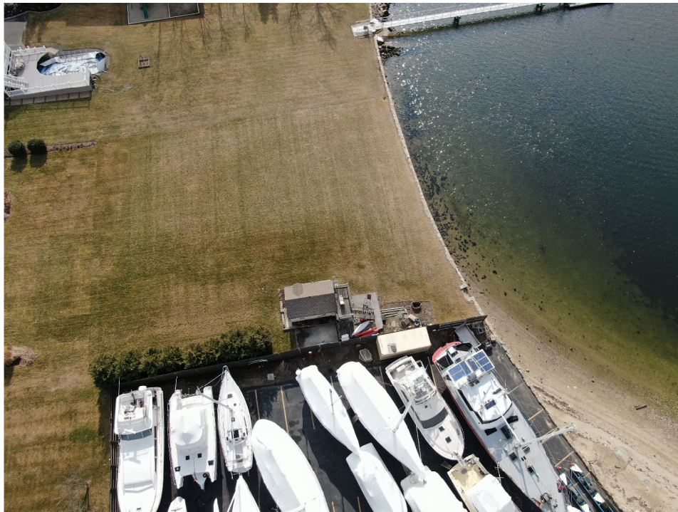
Aerial view of existing project site – 32 Fort St.
