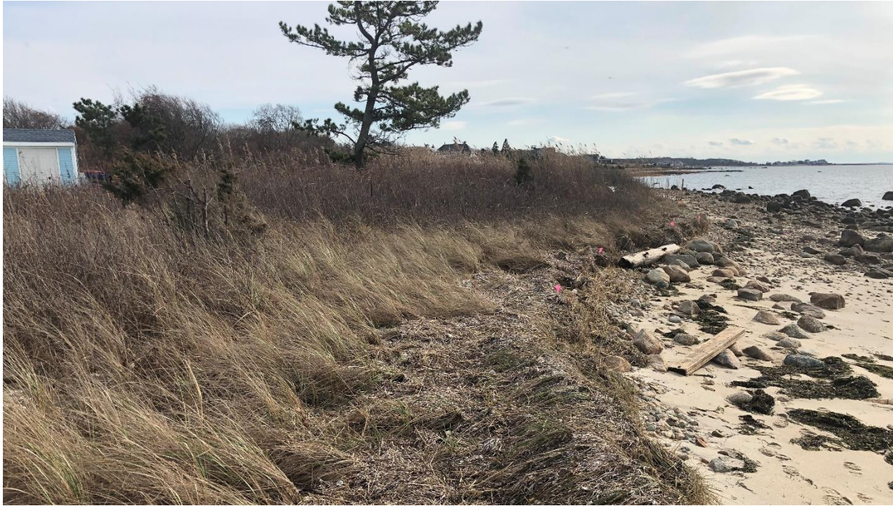
Photo 4. Looking south at the Coastal Dune that lies north of the Jerusalem Road access to the beach. The landward edge of this portion of the Coastal Dune is defined by the edge of lawn at 1 Jerusalem Road.
