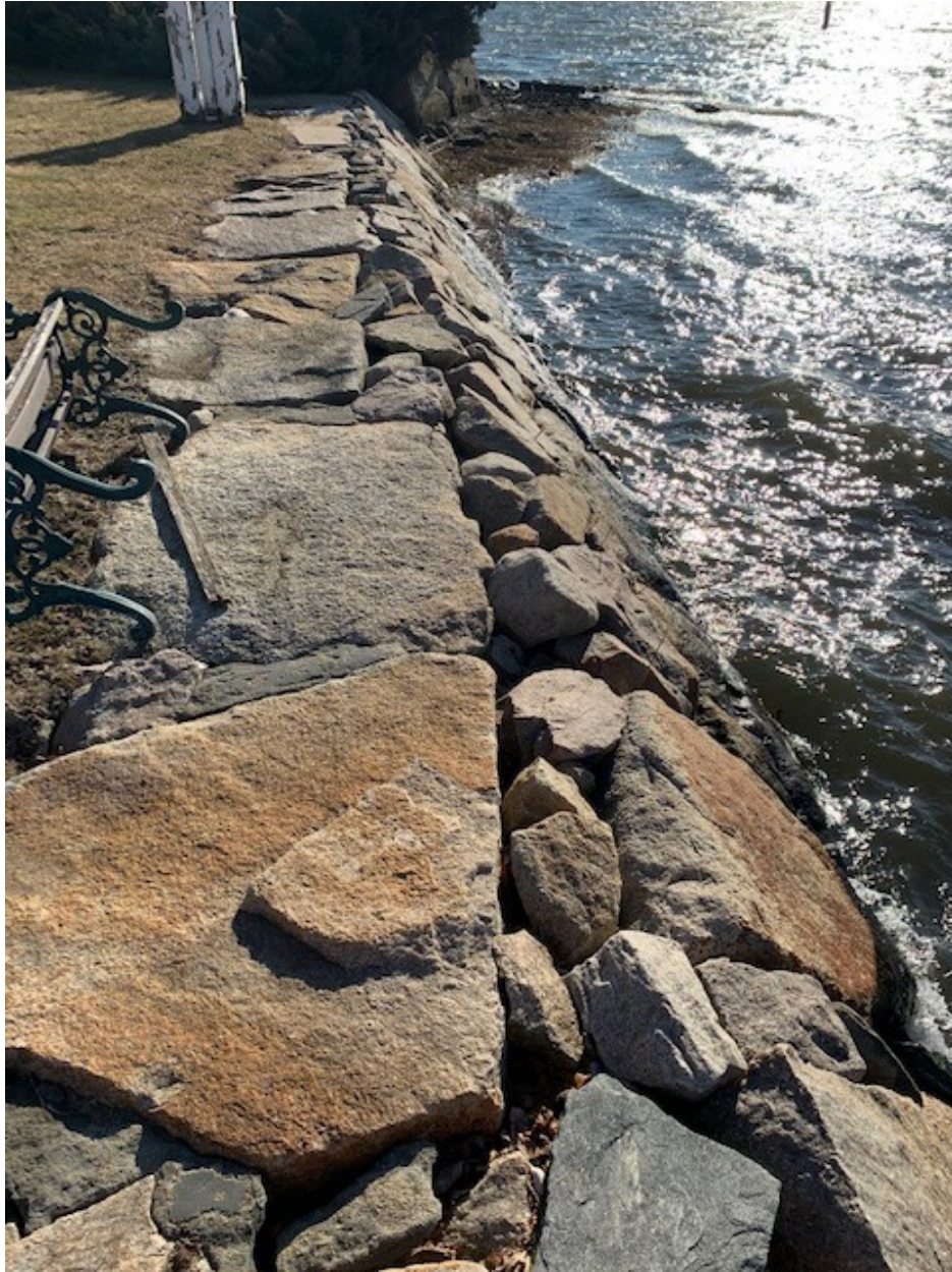
Seawall looking south
