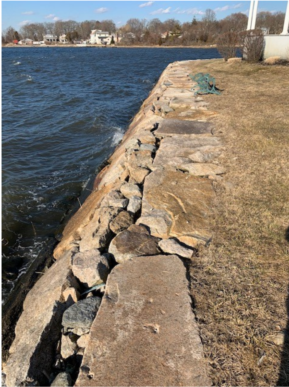
Seawall looking north
