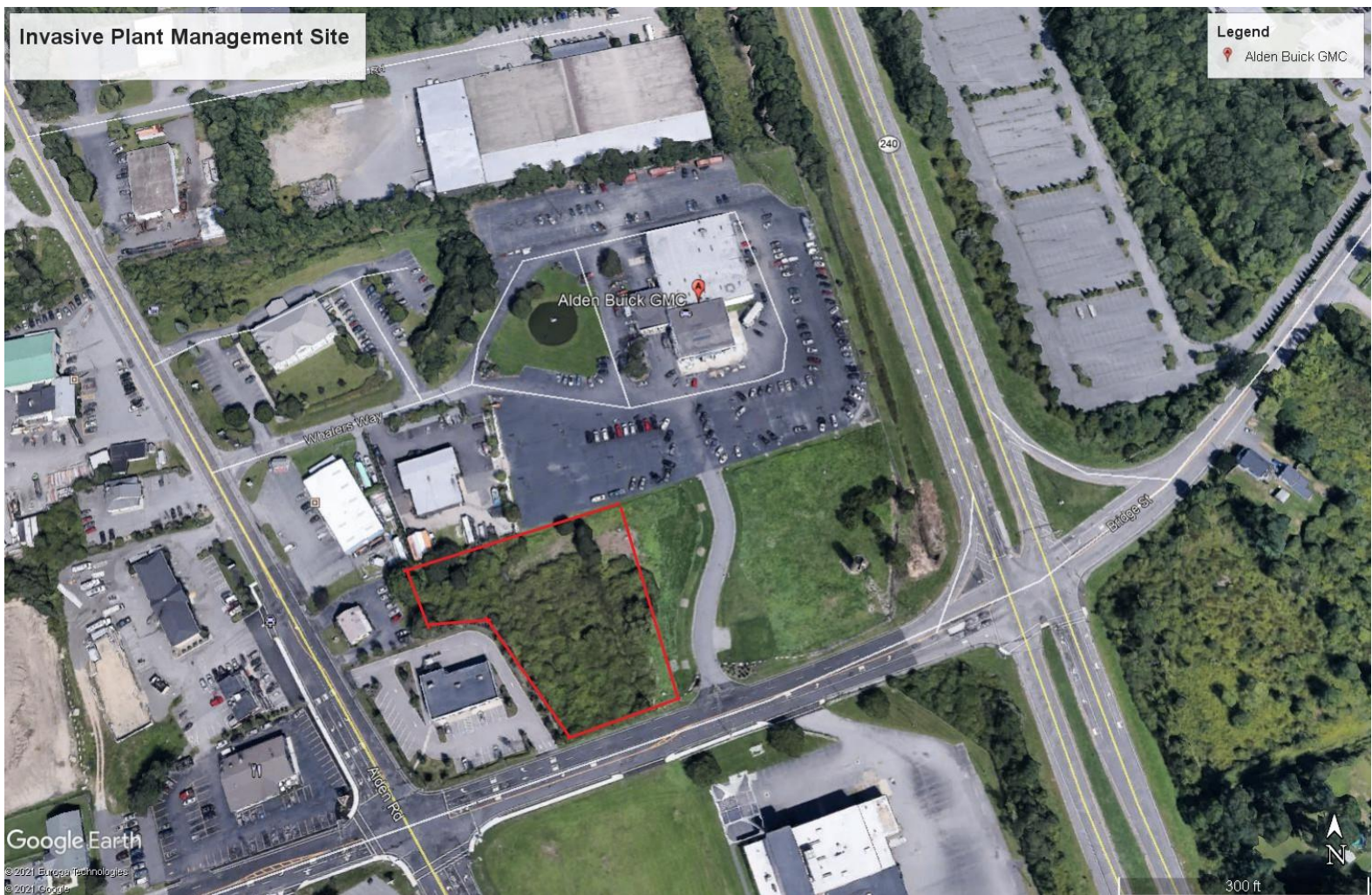
Site aerial view, invasive work area marked in red.
