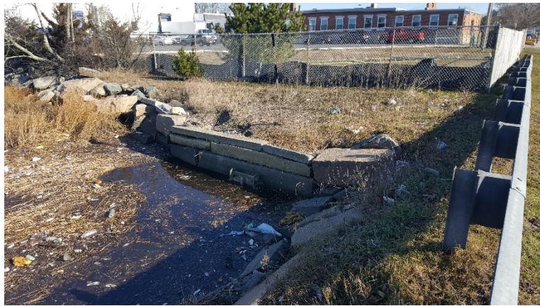
Figure 2: East view of the metal pipe and tide-gate with riprap.
