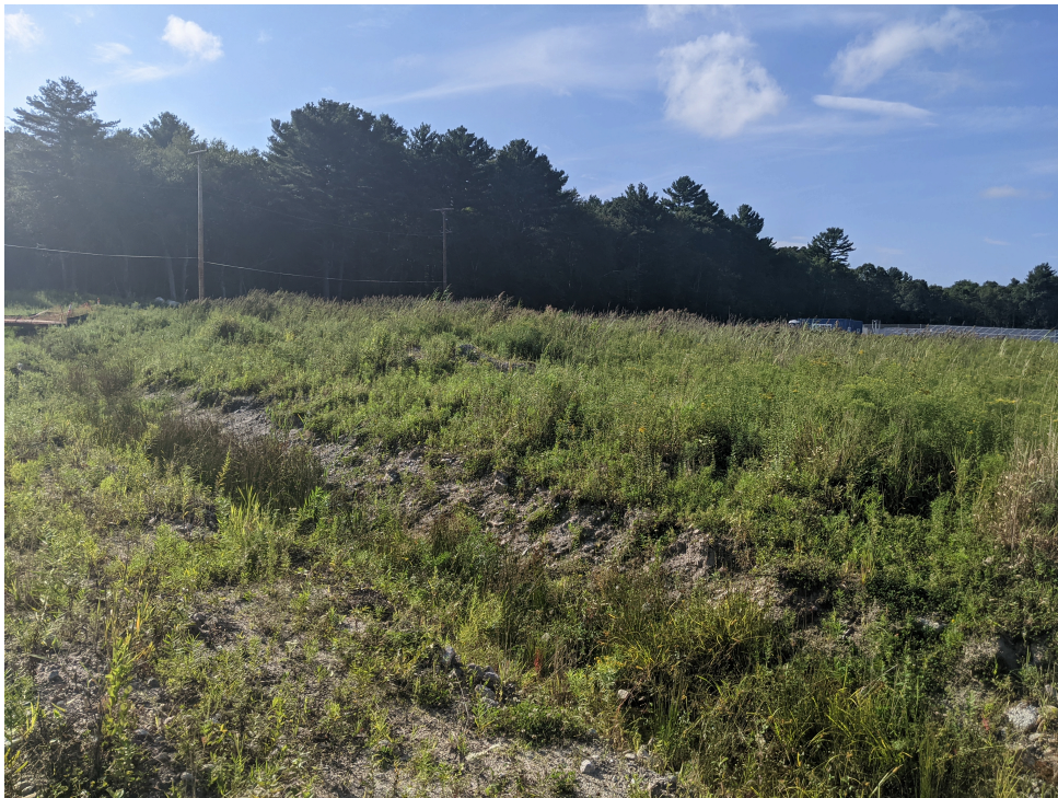
Figure 1. The on-site stream and proposed location of the restoration area. Existing solar panels under construction are shown in the background.
