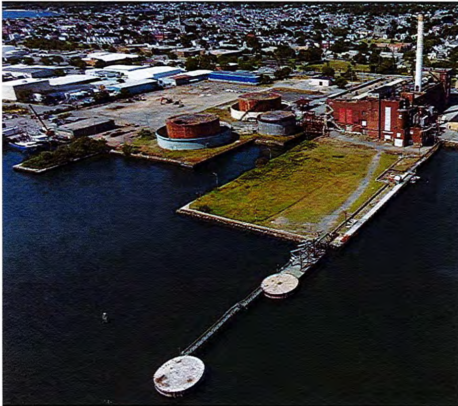
Existing Conditions Photo
