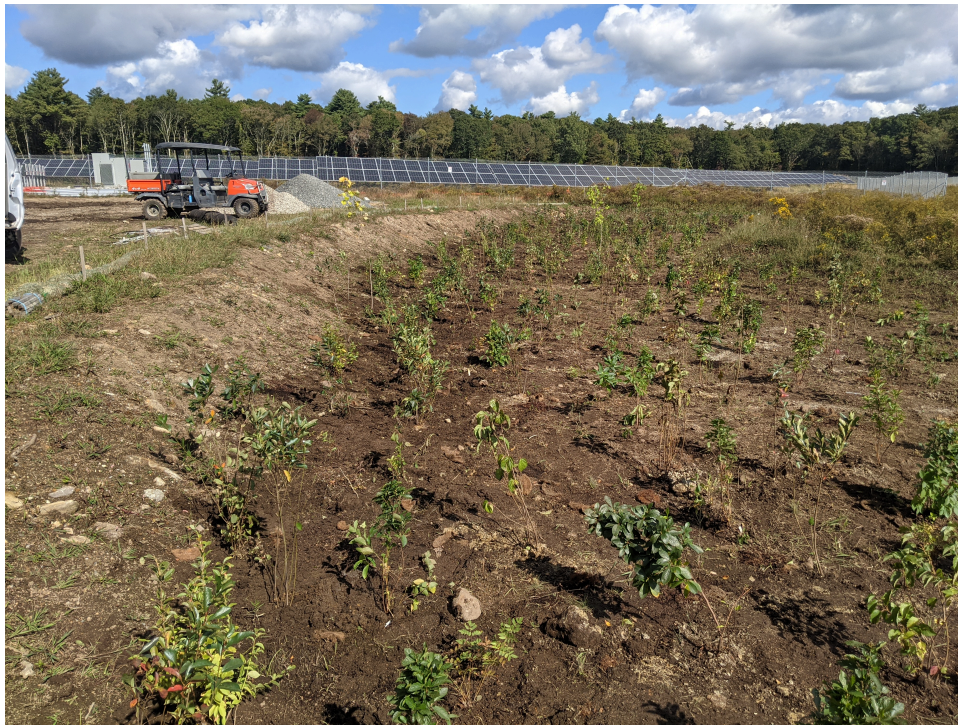
Figure 3. The completed wetland replication area looking north.
