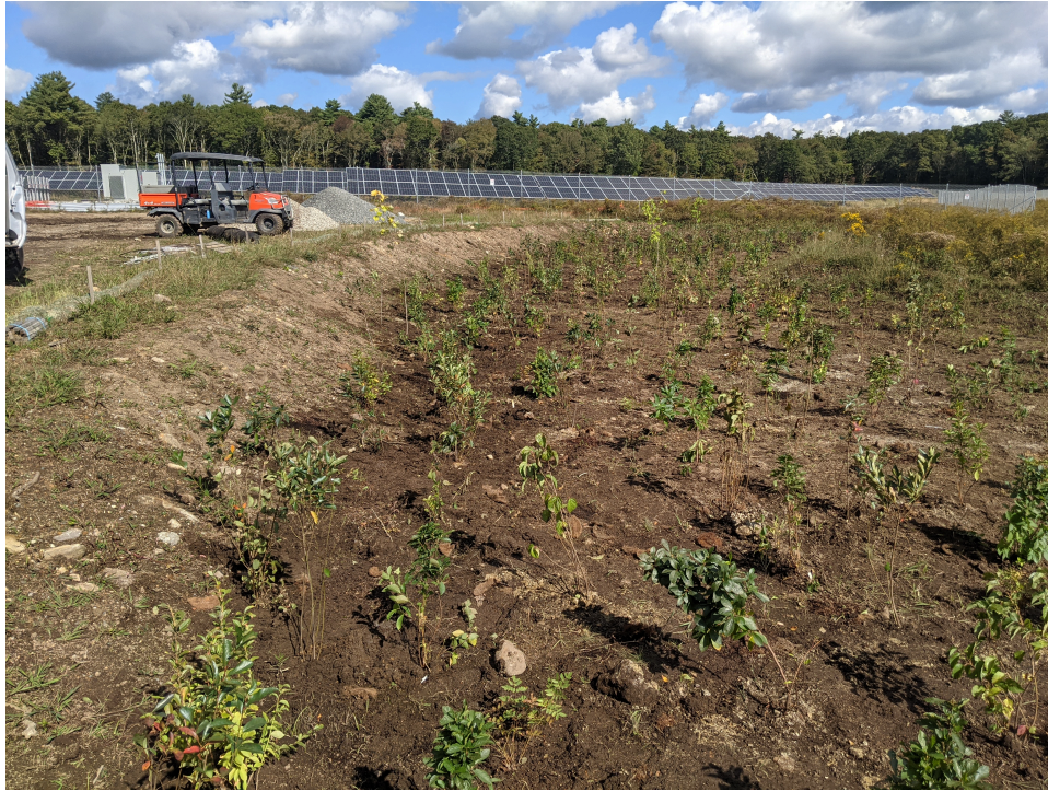
Figure 3. The completed wetland replication area looking north.
