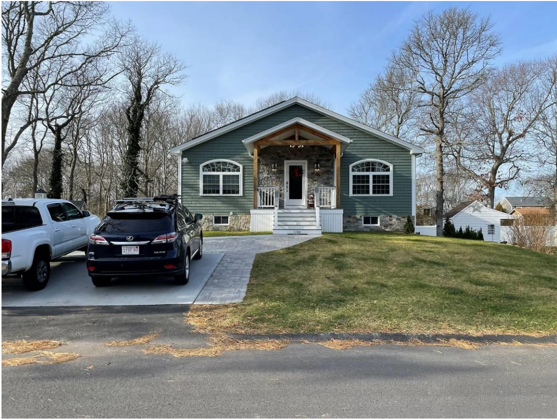
Photograph #1 – View from Ebony Street toward the front of the newly constructed single-family home. The site surrounding the home is fully stabilized.
