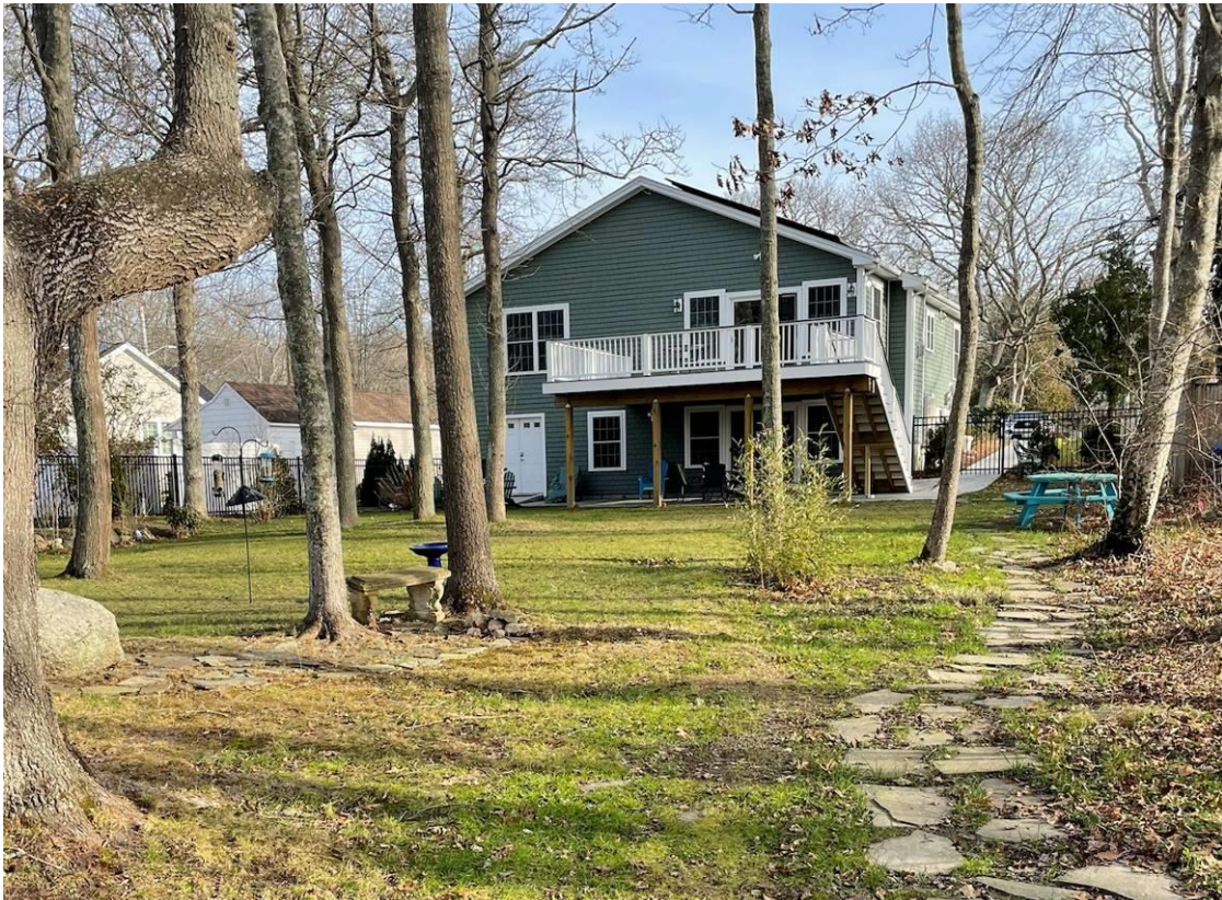
Photograph #2 - View toward the rear of the newly constructed single-family home.
