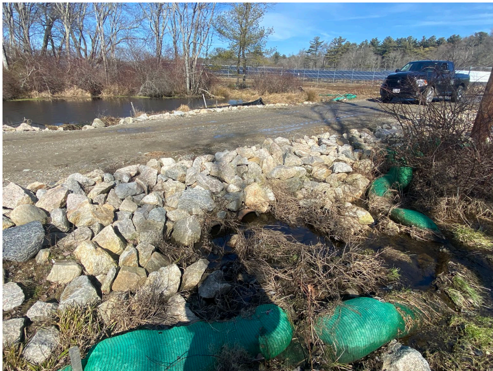
Figure 8: South End of Wetland Crossing "A"
