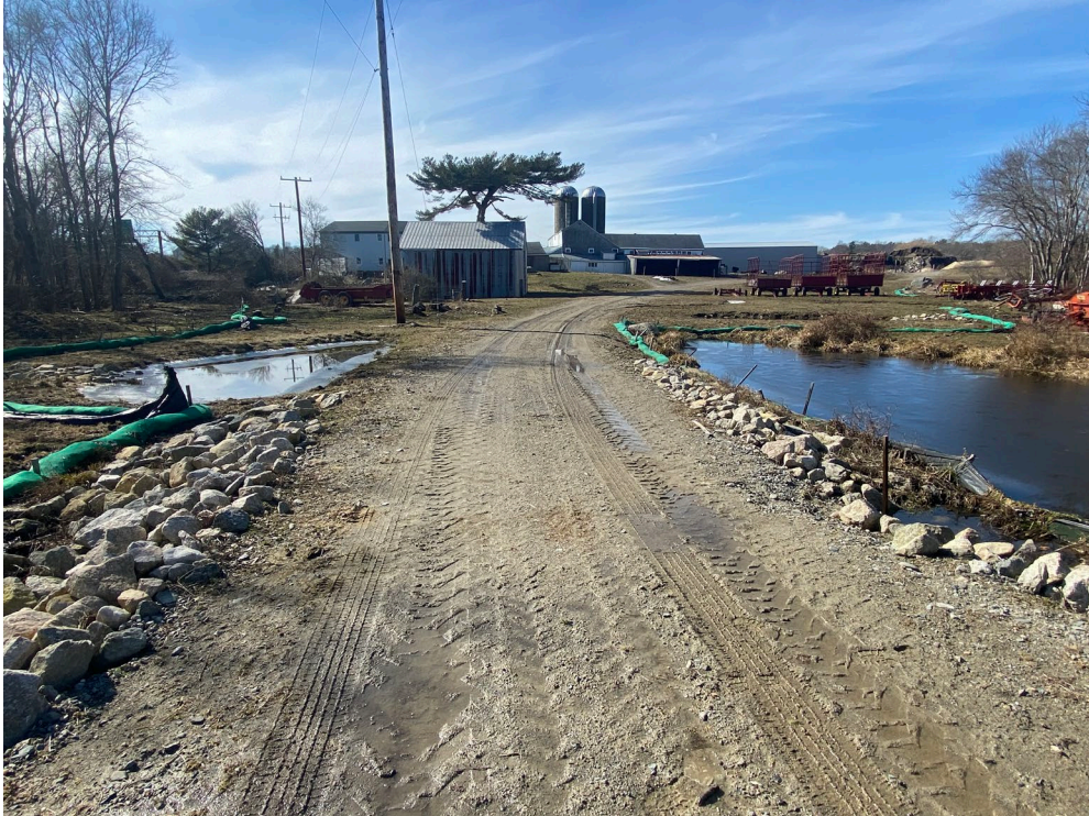
Figure 5: Wetland Crossing "A" West of Main Solar Array
