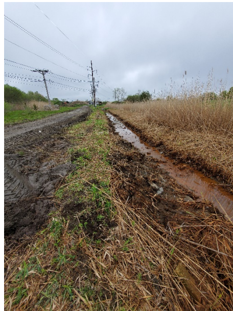
View of drainage swale on westerly abutting landfill property
