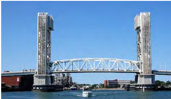
Fore River Bridge
