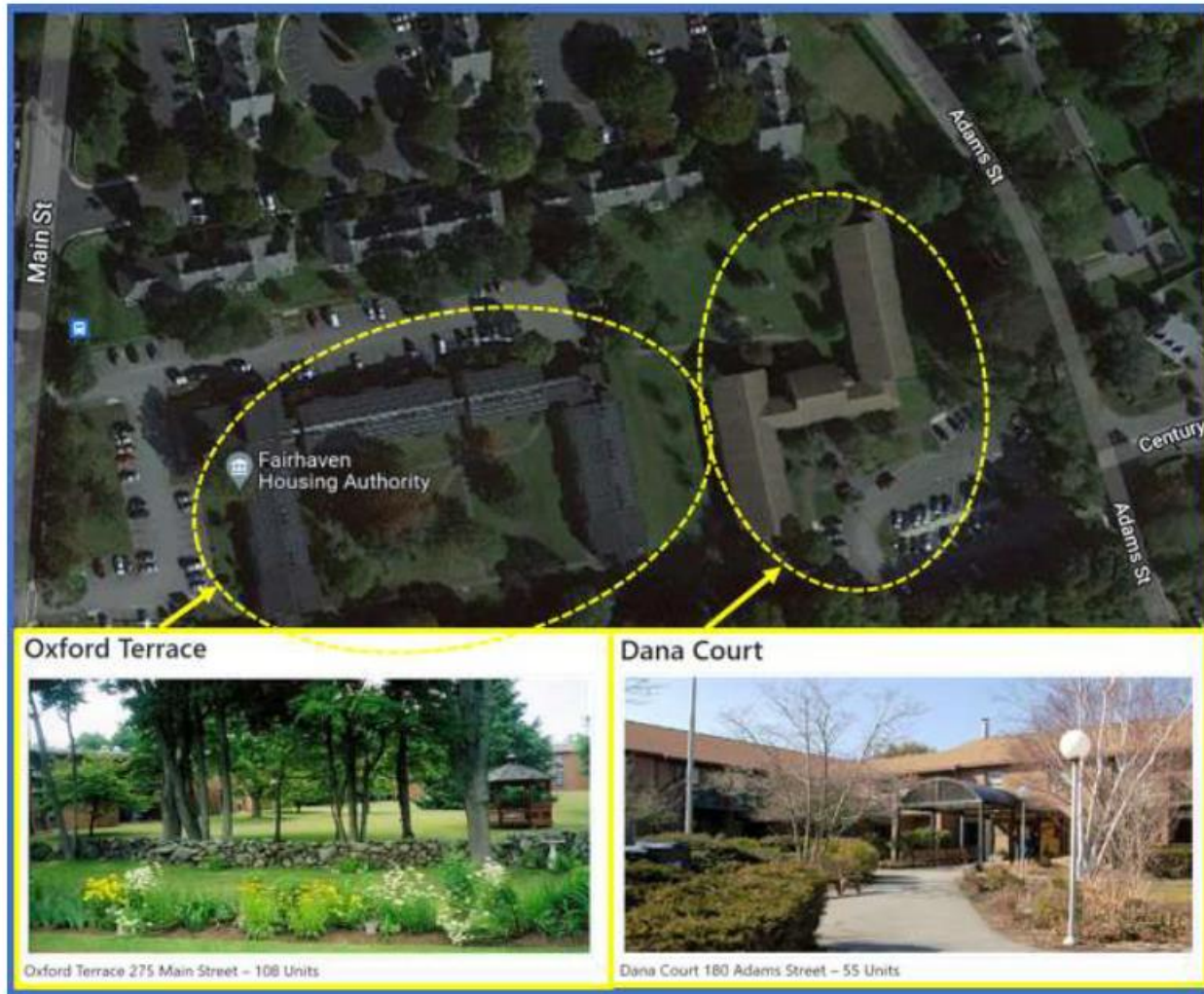
Aerial and site photos.
