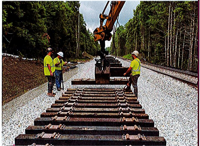
Setting ties on the right of way
