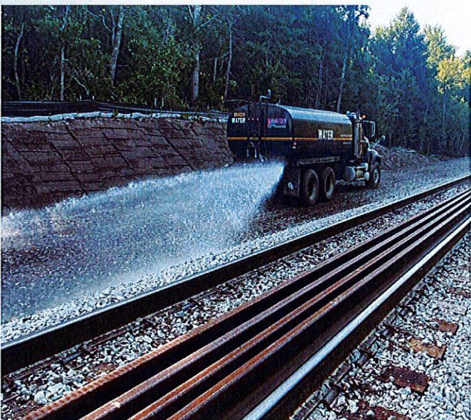
Dust control Cotley Street right of way
