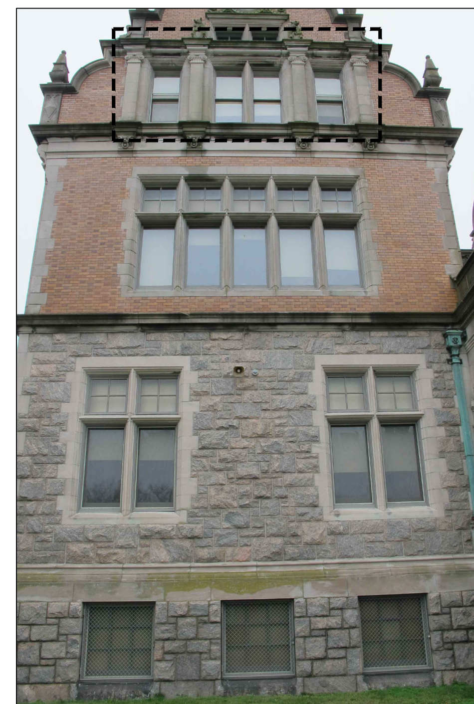
WINDOW TYPE 2 - EXTERIOR DOUBLE-HUNG WINDOW (AREA INDICATED)
