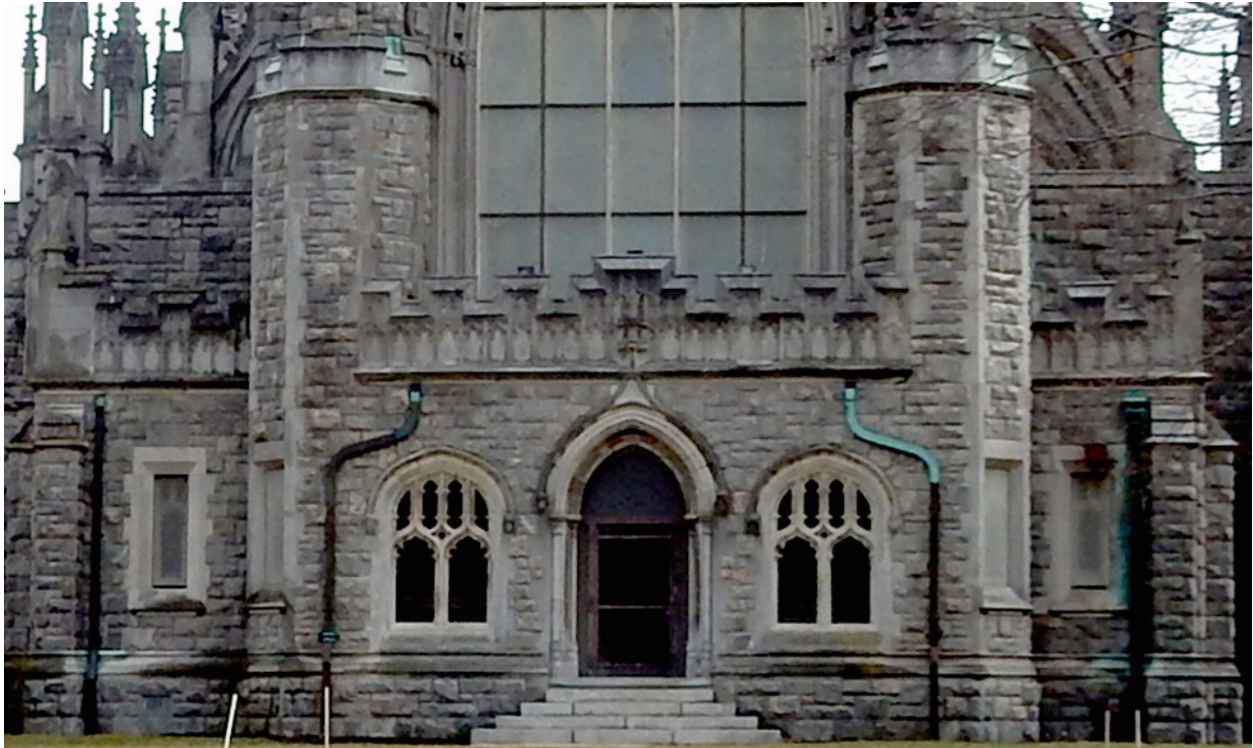
Downspouts and metal box above window.
