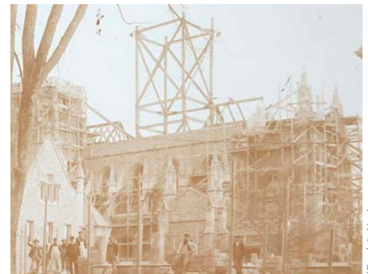
Church Sanctuary under construction.
