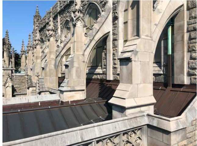
Newer copper replacement roof over west ambulatory and porch.
