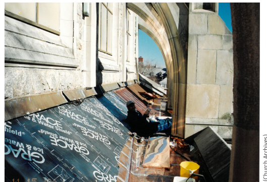
2004 gutter and roof repairs.
