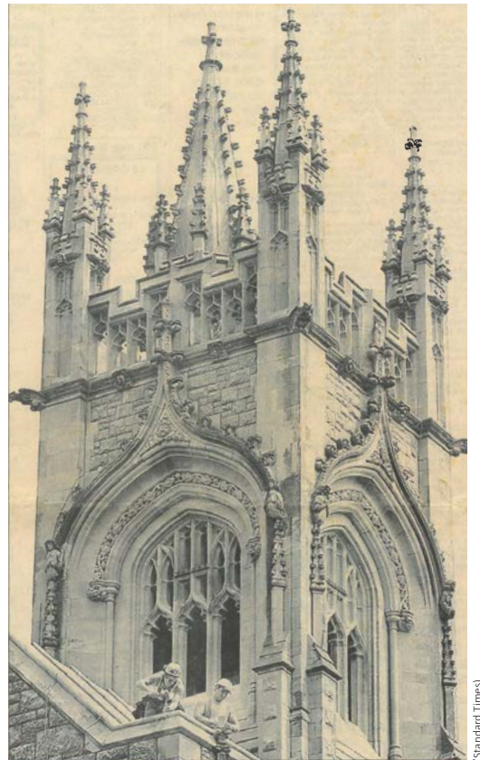
Workers from Flagship Roofing making repairs in 2002.
