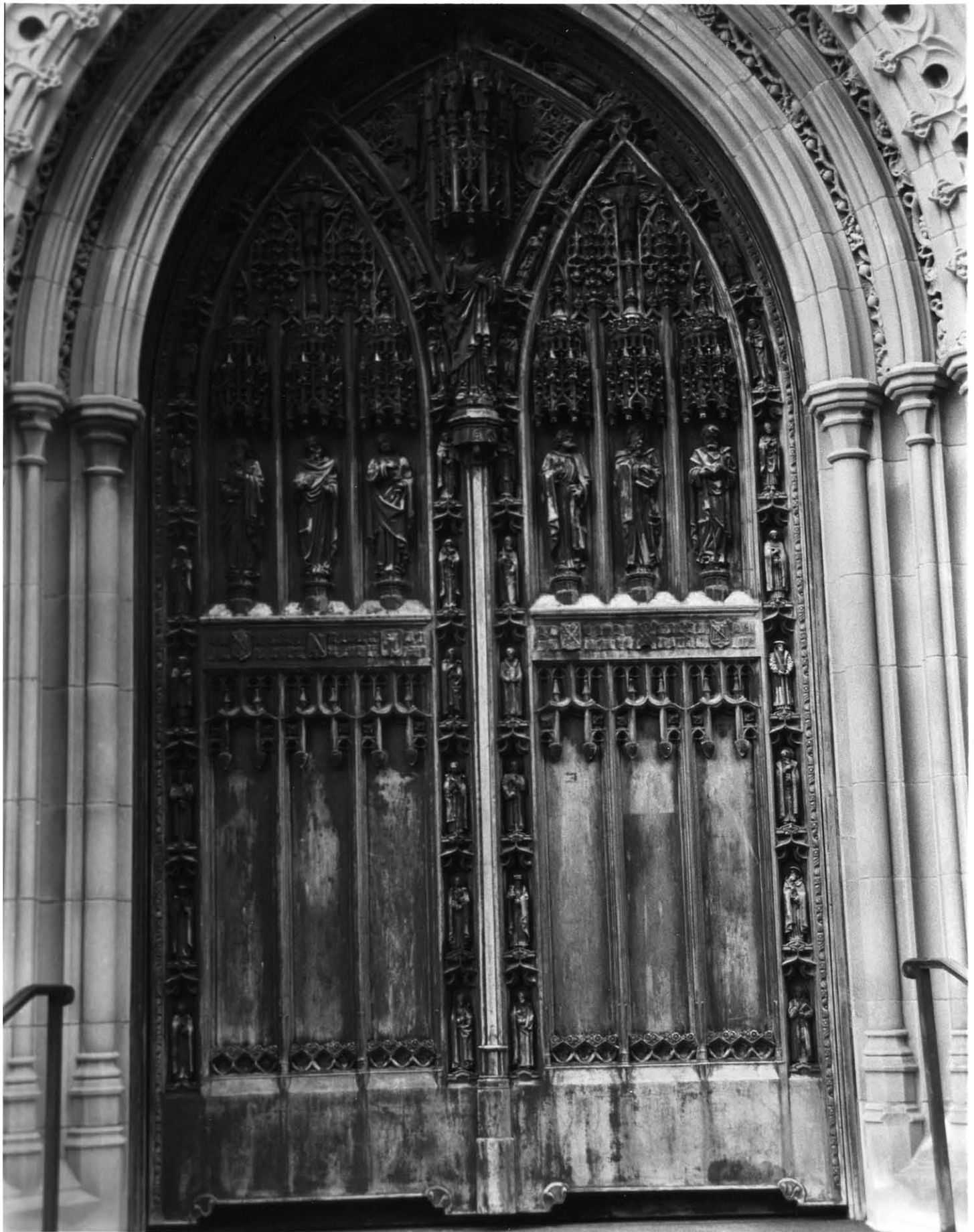
3. Doors to sanctuary, south elevation. (Photograph: Willoughby Elliott, May 1995)
