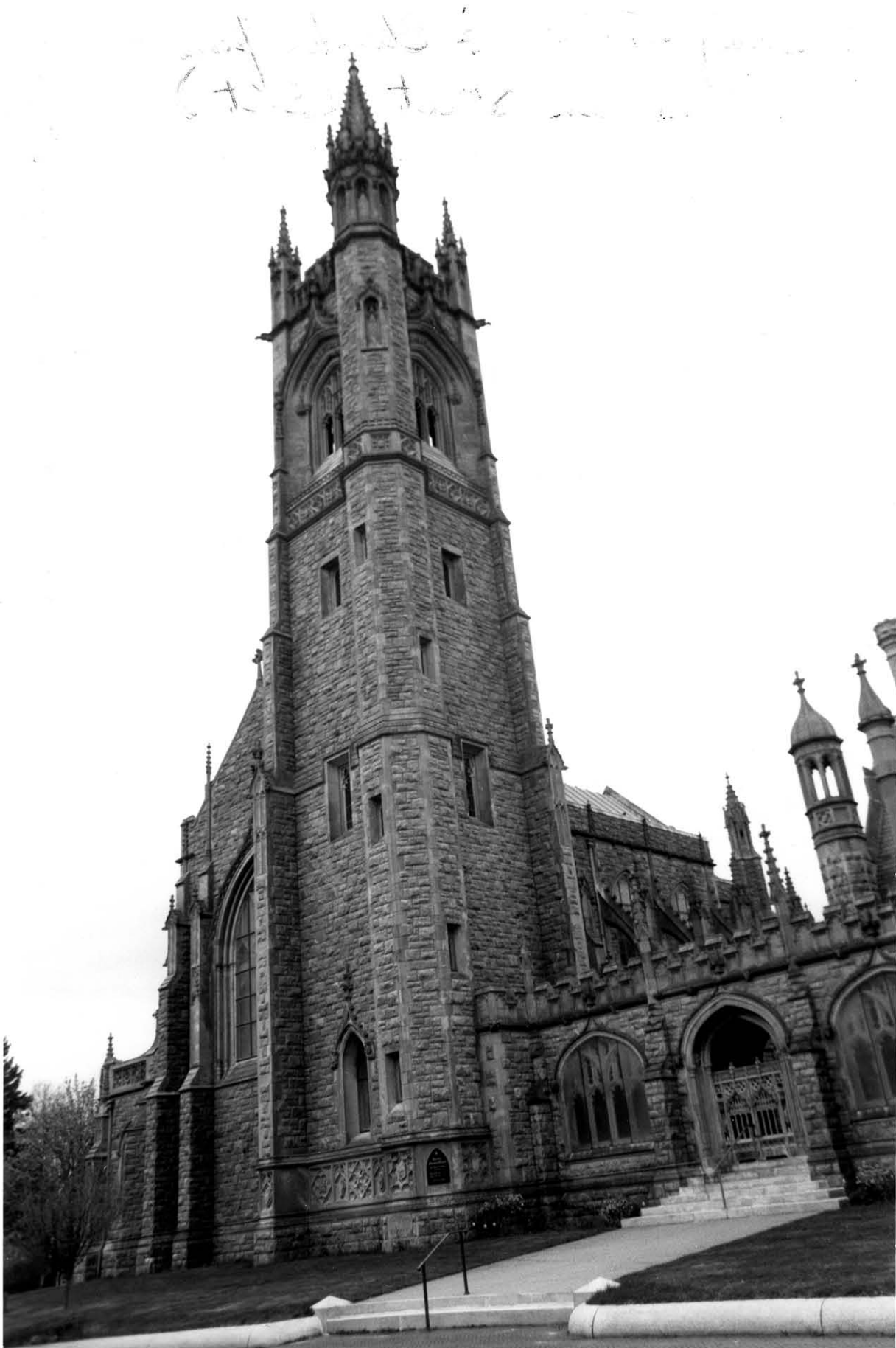
2. Tower from northeast. (Photograph: Willoughby Elliott, May 1995)
