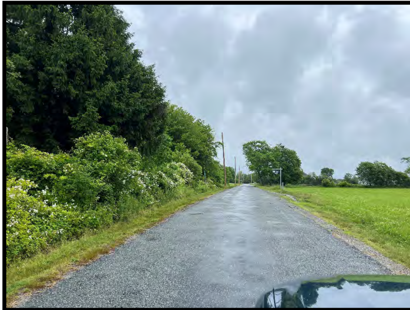
Subject to left facing east on Shaw Road
