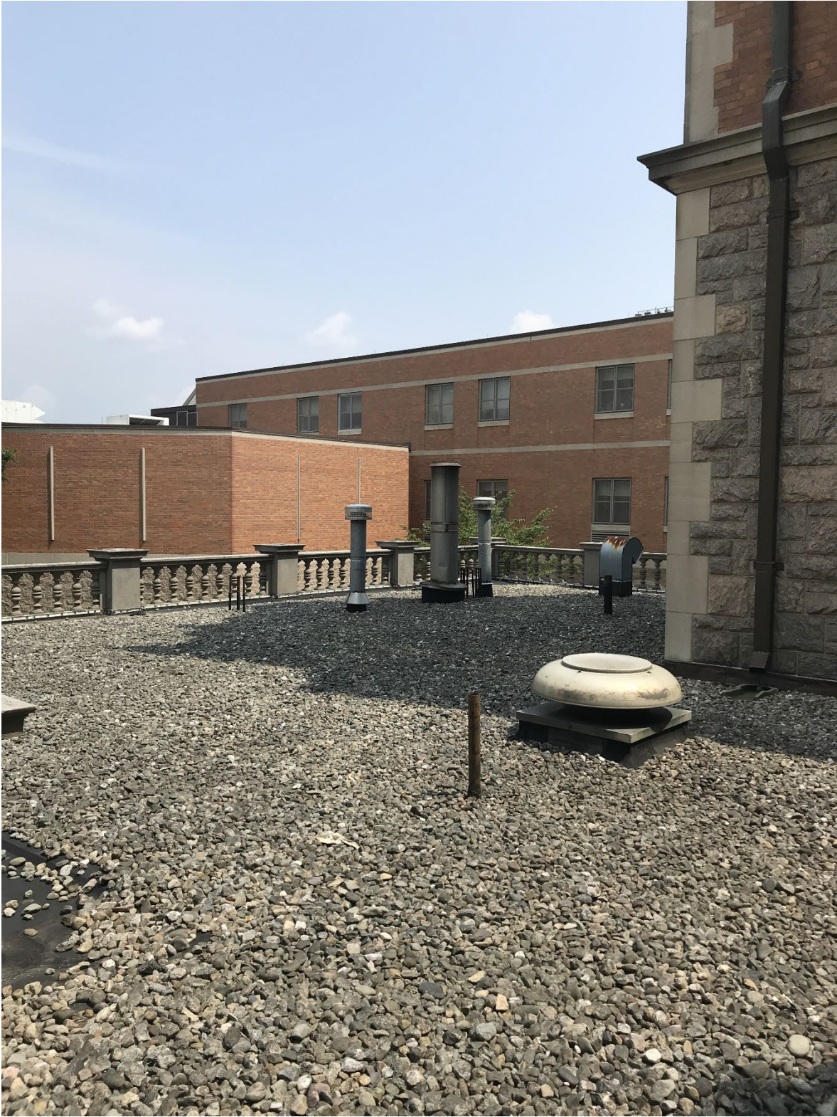
Figure 2 View of the low-pitched roof over the boiler room
