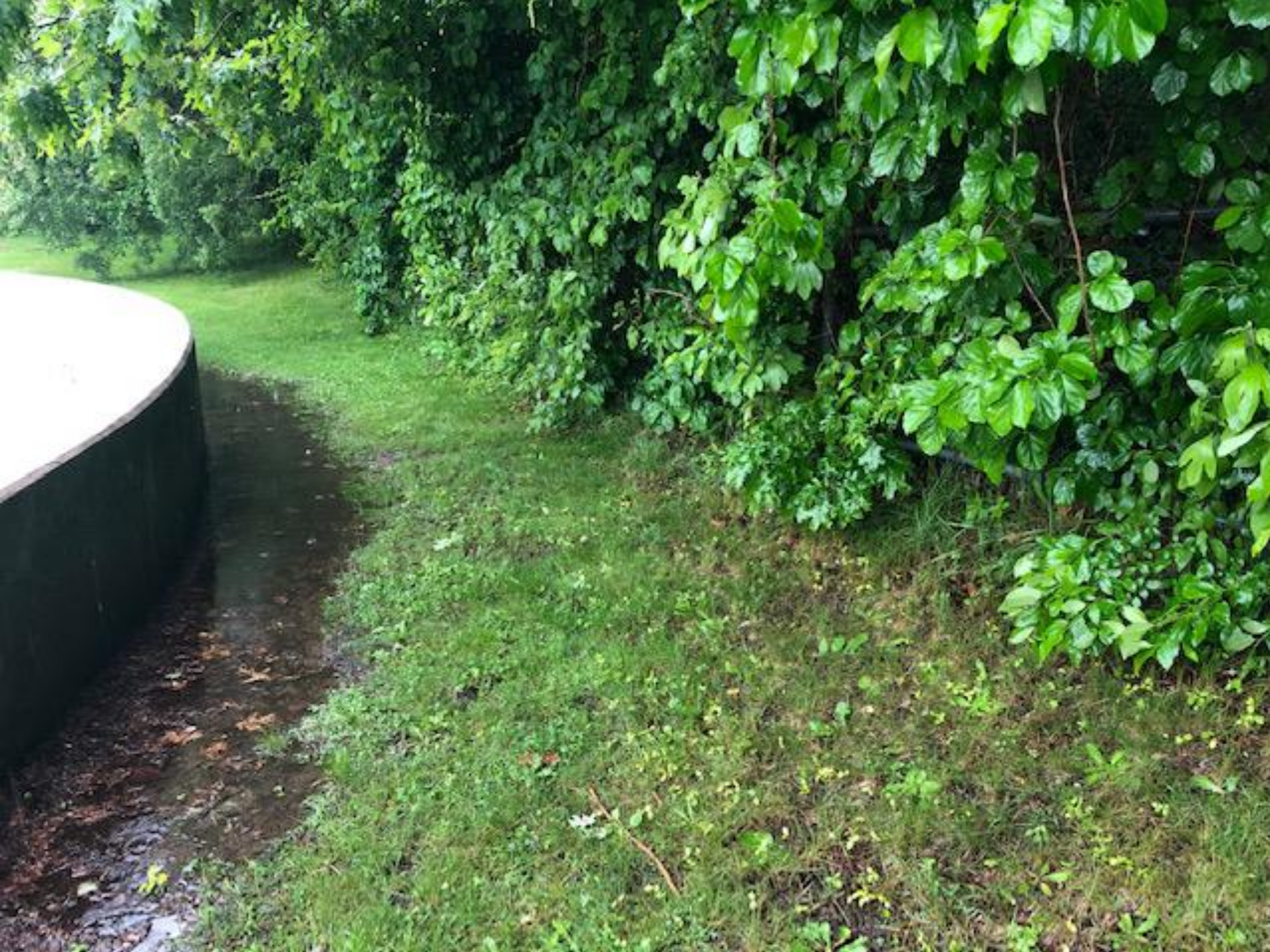
Sewage Treatment Plant Clarifying Pit Near Lot 11
