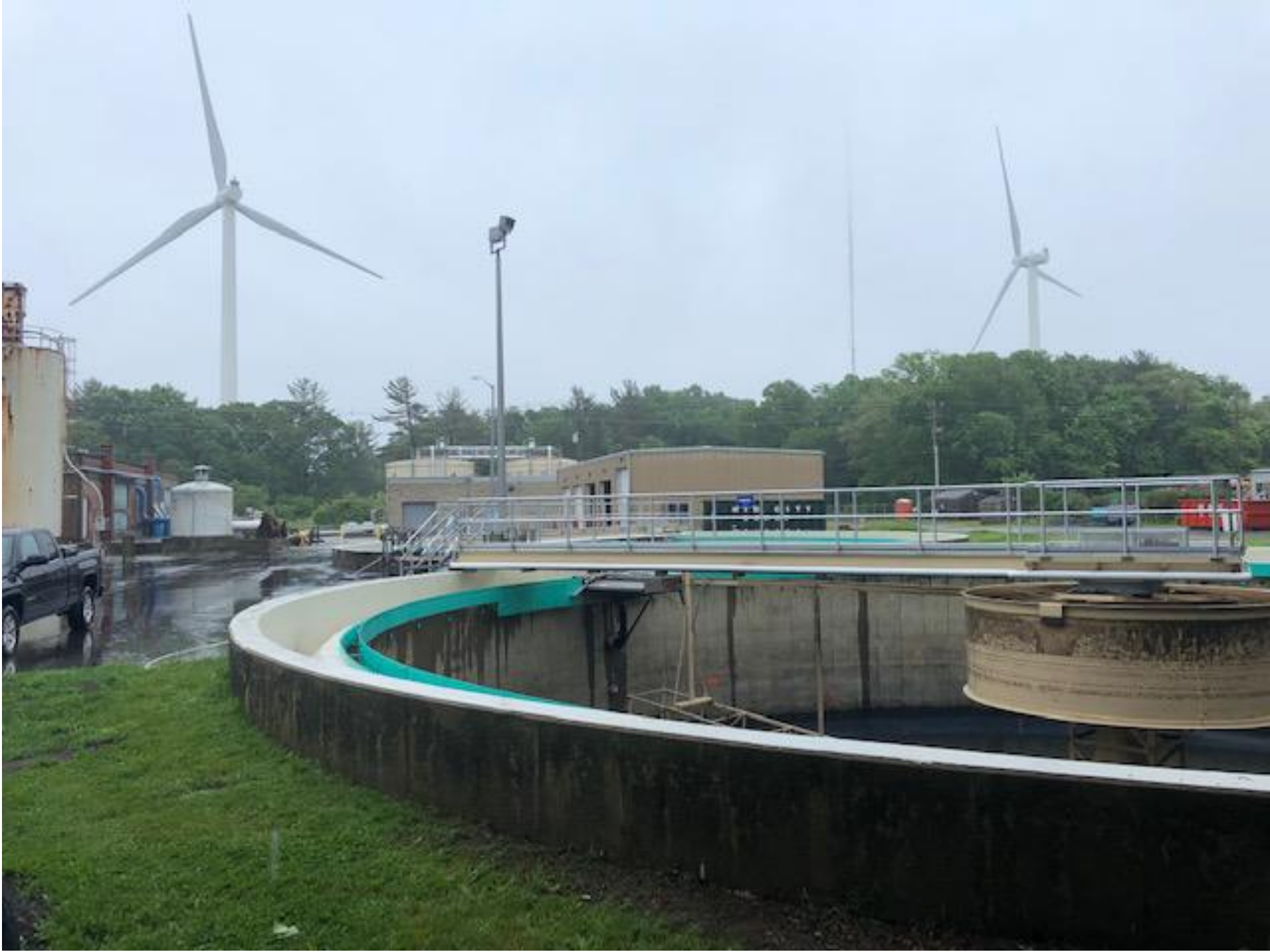
Sewage Treatment Plant & Wind Turbines
