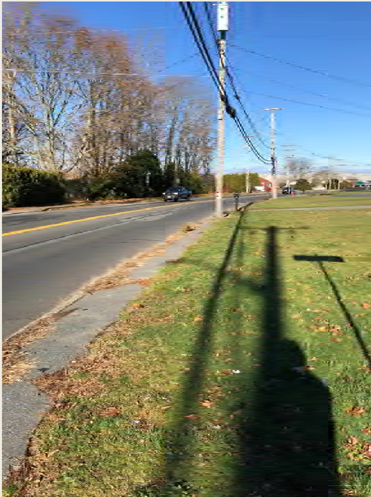
Sidewalk Surface in Below Average Condition on Sconticut Neck Rd at Marilaine Pl
