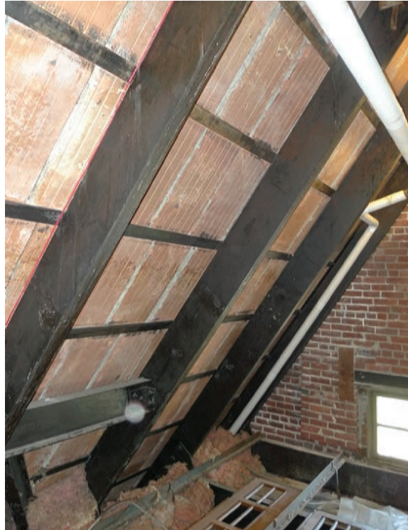
Photograph 5: Existing steel framing at gable windows.
