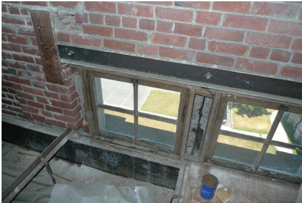
Photograph 6: Closeup of existing steel at gable windows.
