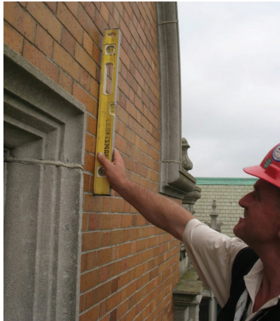
Photograph 3: Existing condition showing inward-leaning masonry.
