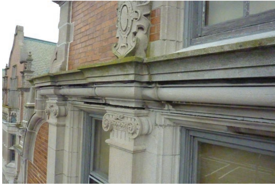
Photograph 1: Existing condition at gable, showing widening cap above pilasters.
