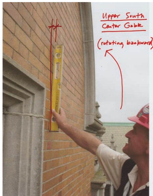
Photograph 4: Same photos as above, showing inward-leaning masonry wall. Note angle of level positioned against masonry wall.
