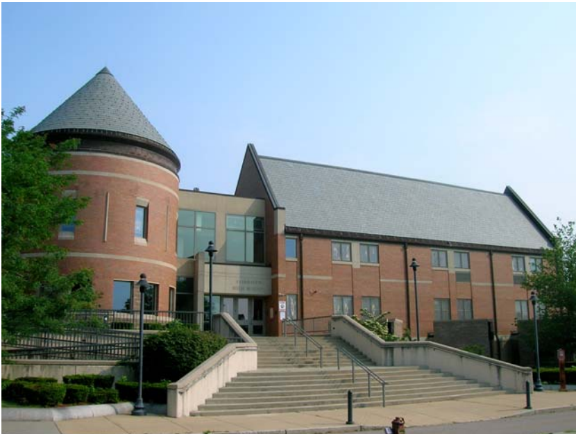
View of the 1996 Addition
