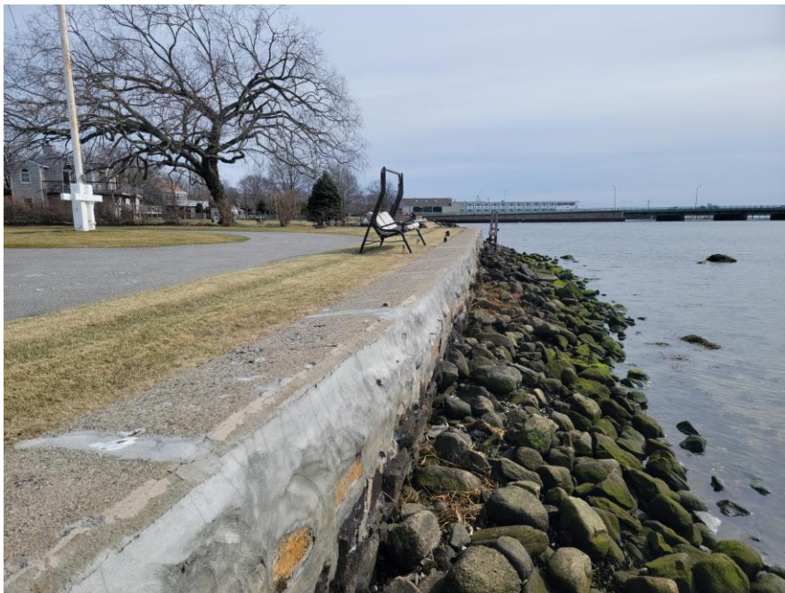
Photo 4 – 8 Winslow Court – Seawall/RipRap – Facing South
