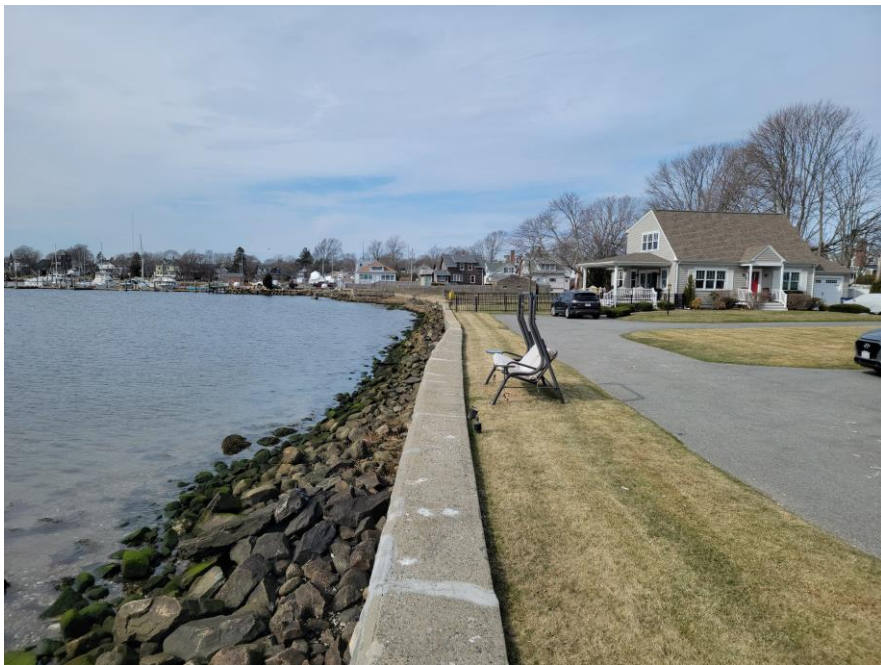
Photo 2 – 8 Winslow Court – Seawall Facing North
