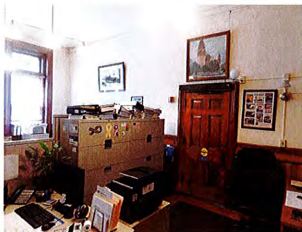
Door from Elevator platform into Assessor's Office. Note power operator on top of door.
