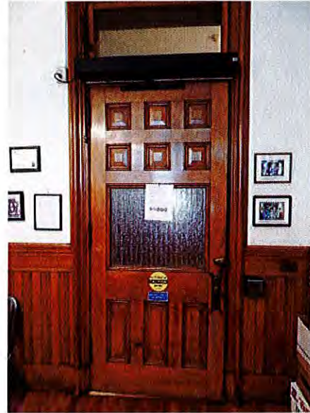
Door from Assessor's Office to upper corridor, leading to the Main office and Building Department
