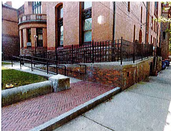
Exterior Ramp at Northeast corner of Town Hall
