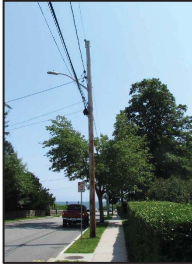
Figure 1: Existing Utility Pole at 6 Fort Street, Fairhaven, MA Which Would Host a Verizon Wireless SC Antenna
